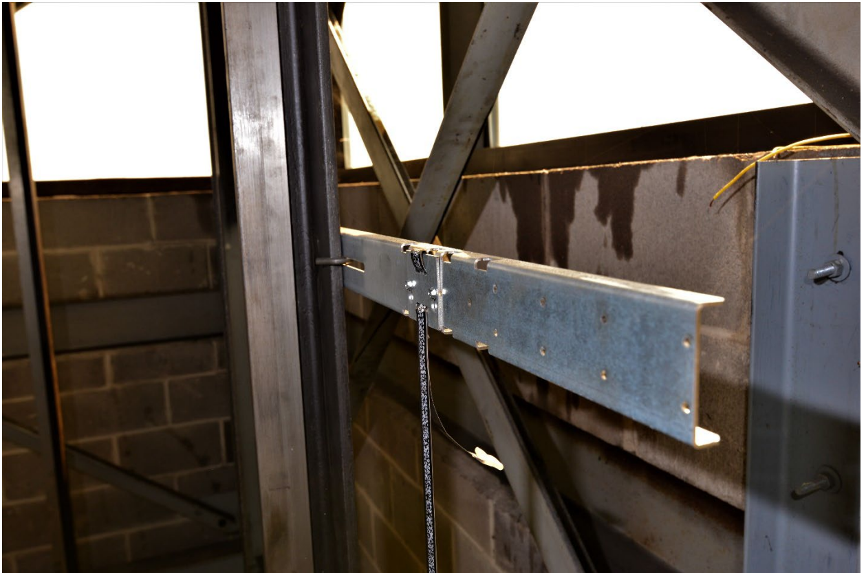
Figure E1.1: Top Tape Bracket
